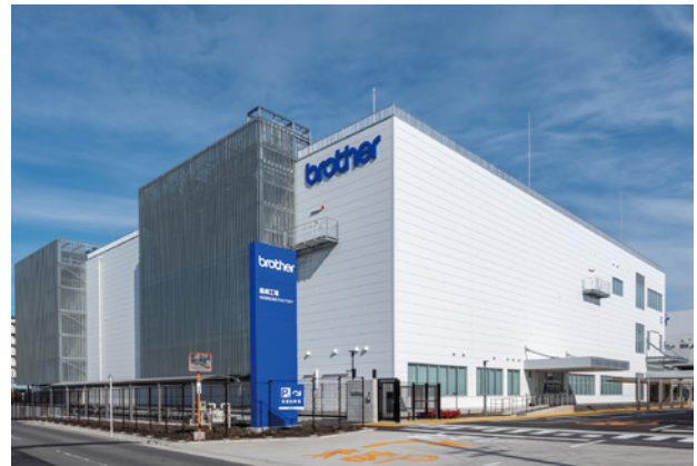
Completed Hoshizaki Plant No. 13
