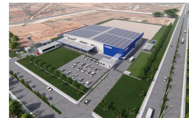
Image of the exterior of the new plant in India
