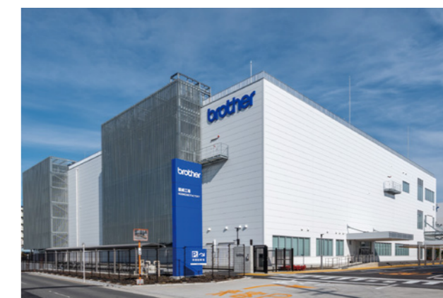
Completed Hoshizaki Plant No. 13
