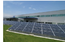
Solar panel in Kariya Factory
