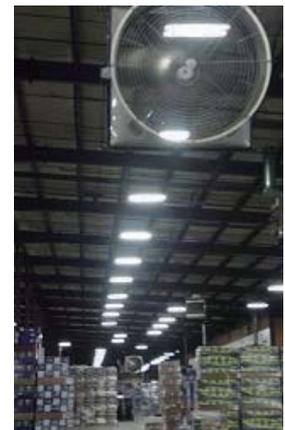
In the warehouse area, extra-large fans were fixed to the ceiling to keep employees cooler in summer. In winter, warm air is circulated on the floor surface to increase the heating efficiency and reduce fuel consumed by the boiler. In FY2015, the energy consumption was reduced by about 580 MWh from FY2014.
