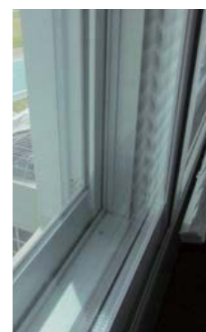
Double-pane glass window sashes (interior side of windows)
