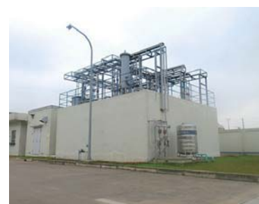
Wastewater treatment facility (BMV)
