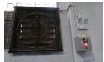
Temperature sensor for activating an exhaust fan when the temperature is 35°C or higher
