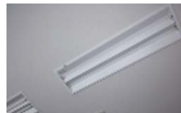
Removing fluorescent lights where possible
