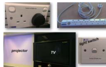
Fully observing the rule to switch off the equipment
