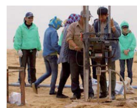
Drilling a well using a drilling machine
