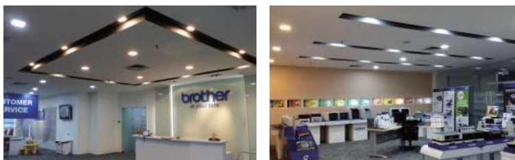
LED lamps used in the showroom and service center
