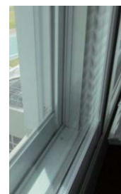
Double-pane glass window sashes (interior side of windows)
