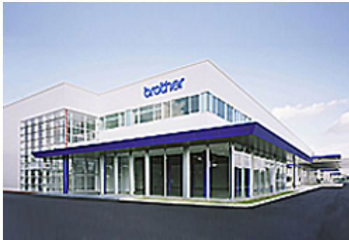
M&S Kariya Plant
