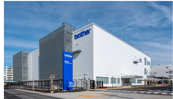
New factory building of Hoshizaki Factory (Factory No. 13)
