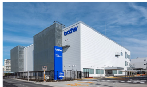
New factory building of Hoshizaki Factory (Factory No. 13)
